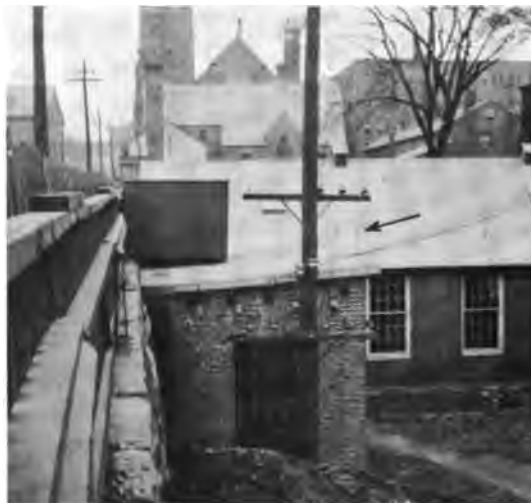
Fig. 4. Accident on Roof.
